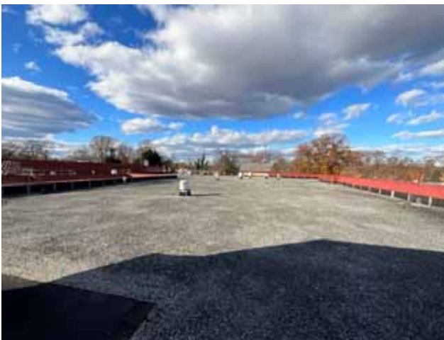
29 - PRIMARY ROOF OVERVIEW
