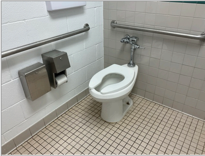
TOILET STALL OVERVIEW
